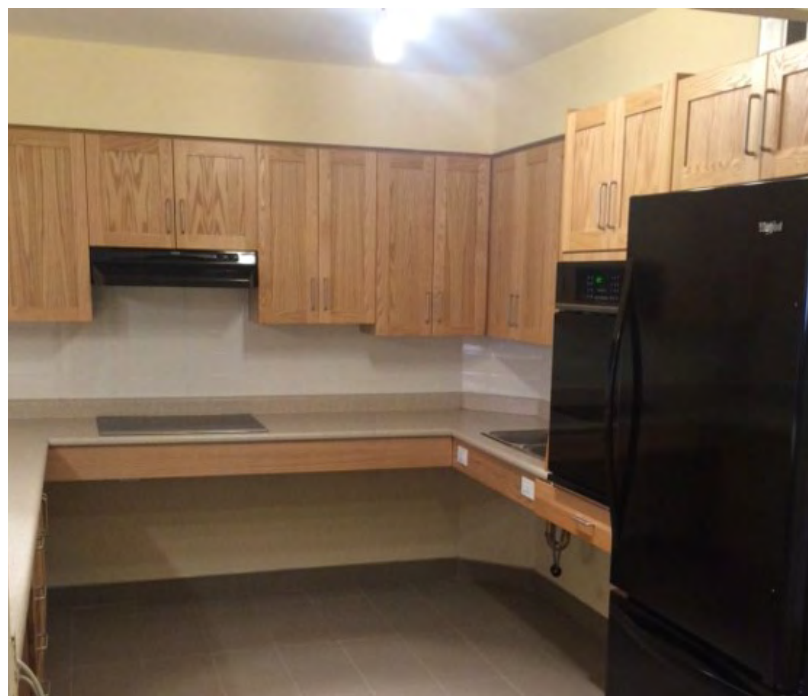
Kitchen modification showing lowered counter in a U shape, there are no cupboards underneath. A wheelchair user will be able to use all parts of the counter. There is a sink and a cooktop mounted on the counter.
